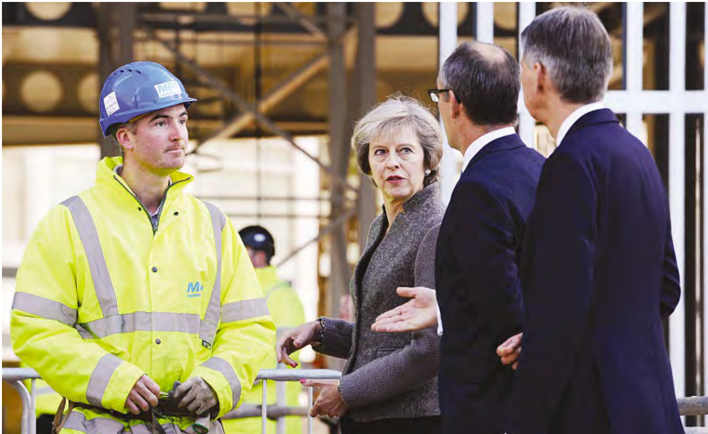
Work in progress: UK prime minister Theresa May visits the Birmingham construction site where HSBC's offices are being built
